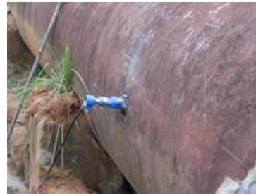
Installation Drawing of Insertion Flow Transducer
