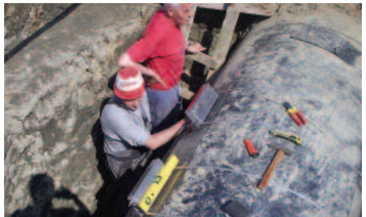
Underground, submersible installation for 56 inch (1425 mm) pipe.
